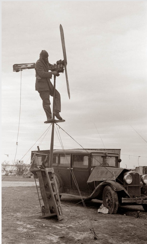
Rural Electrification in the US: Farmers constructed small wind electric plants from Ford's Model T parts using popular manuals (1924-1942)
